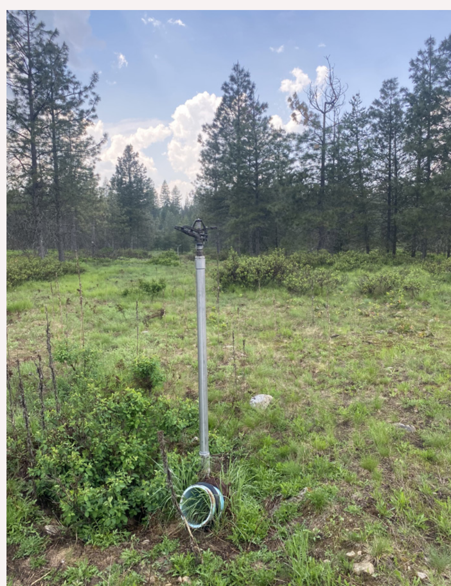
Sprinkler at the Reuse Site
